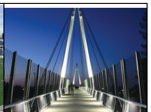
Mary Ave Bicycle Footbridge, Cupertino CA
