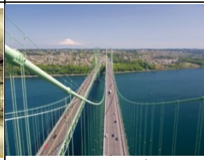
Tacoma Narrows Bridge
