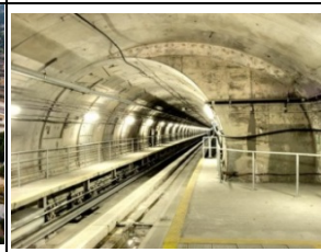
Washington Dulles International Airport Tunnel
