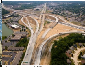
Interstate 465 Reconstruction, Indiana
